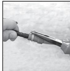
6. Connect the new drain hose to the waste Water pipe.
