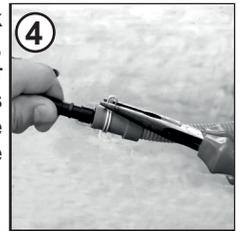
5. Connect the new drain hose to the waste Water pipe.
